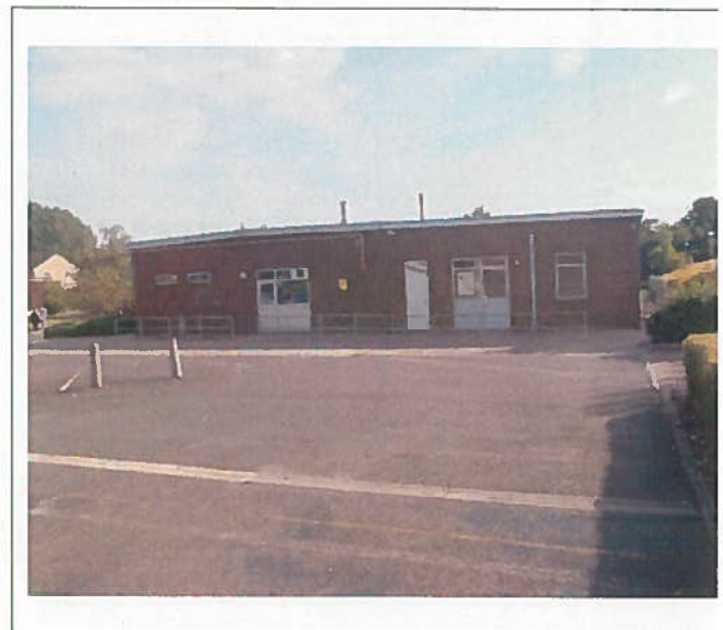
Car park – northern side
